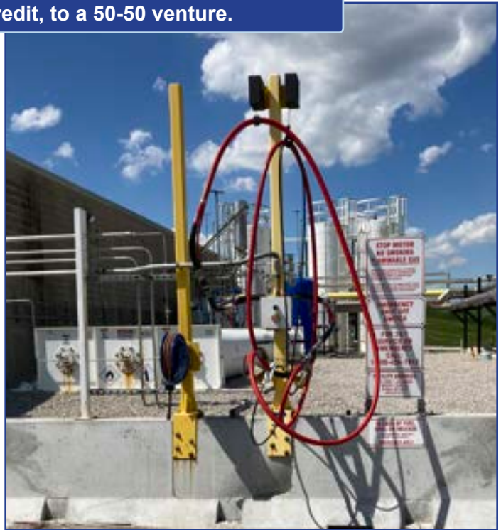
Top: Holding tanks for RNG awaiting transport; Left: Biodigester digestate by-product for cow bedding; Right: Transfer station to load trucks for RNG transport to injection site
