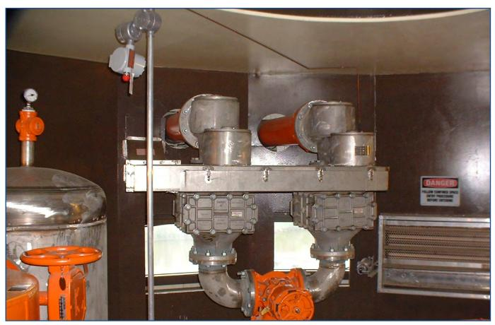
Photo 10: Gas pressure reducing regulator, Appleton Wastewater Treatment Plant
