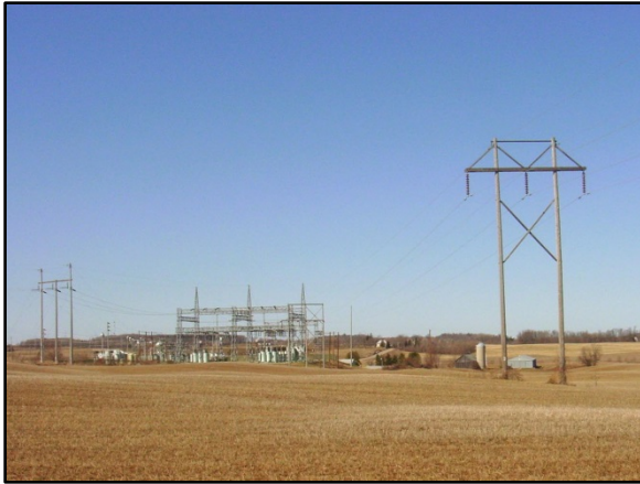
Figure 1 A Variety of Substations in Different Settings
