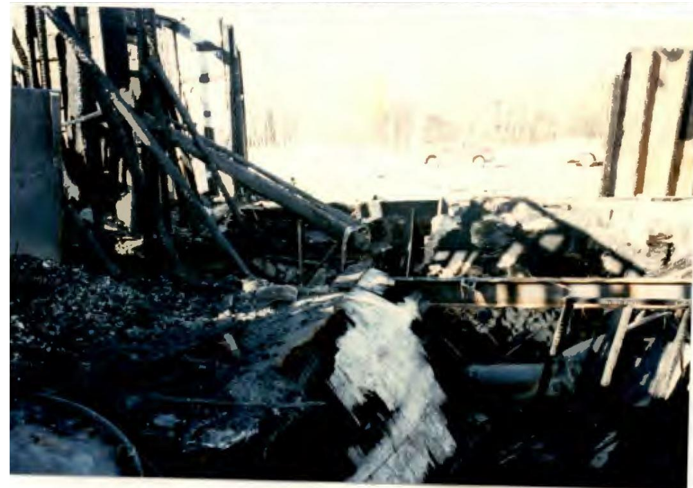
FLOOR OF KITCHEN/DINING AREA
