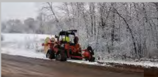
Above: Plowing in mainline fiber in Burnett County with CARES funding
