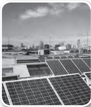
**Solar photovoltaic** uses sunlight to generate electricity to displace energy normally purchased from the electric grid, or to add energy to the electric grid. A map of solar intensity across the United States Wisconsin can be found in the Map Appendix.
