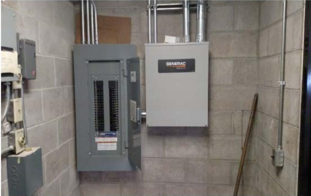
*Backup Power Electrical Panel, right, and RTS Automatic Transfer Switch*
