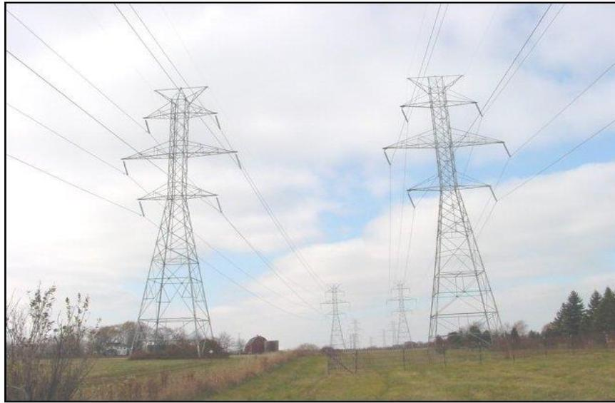
**Figure 3 A Single-Pole, Double-Circuit Transmission Structure**
