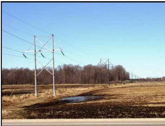
**Figure 2 Typical Single-Pole, Double-Circuit Structure**
