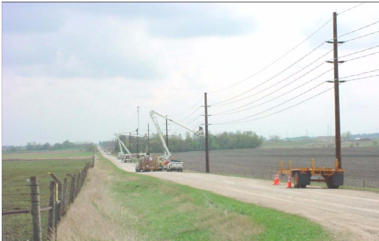
Figure 2-6 Construction of a typical 34.5 kV overhead collector line
