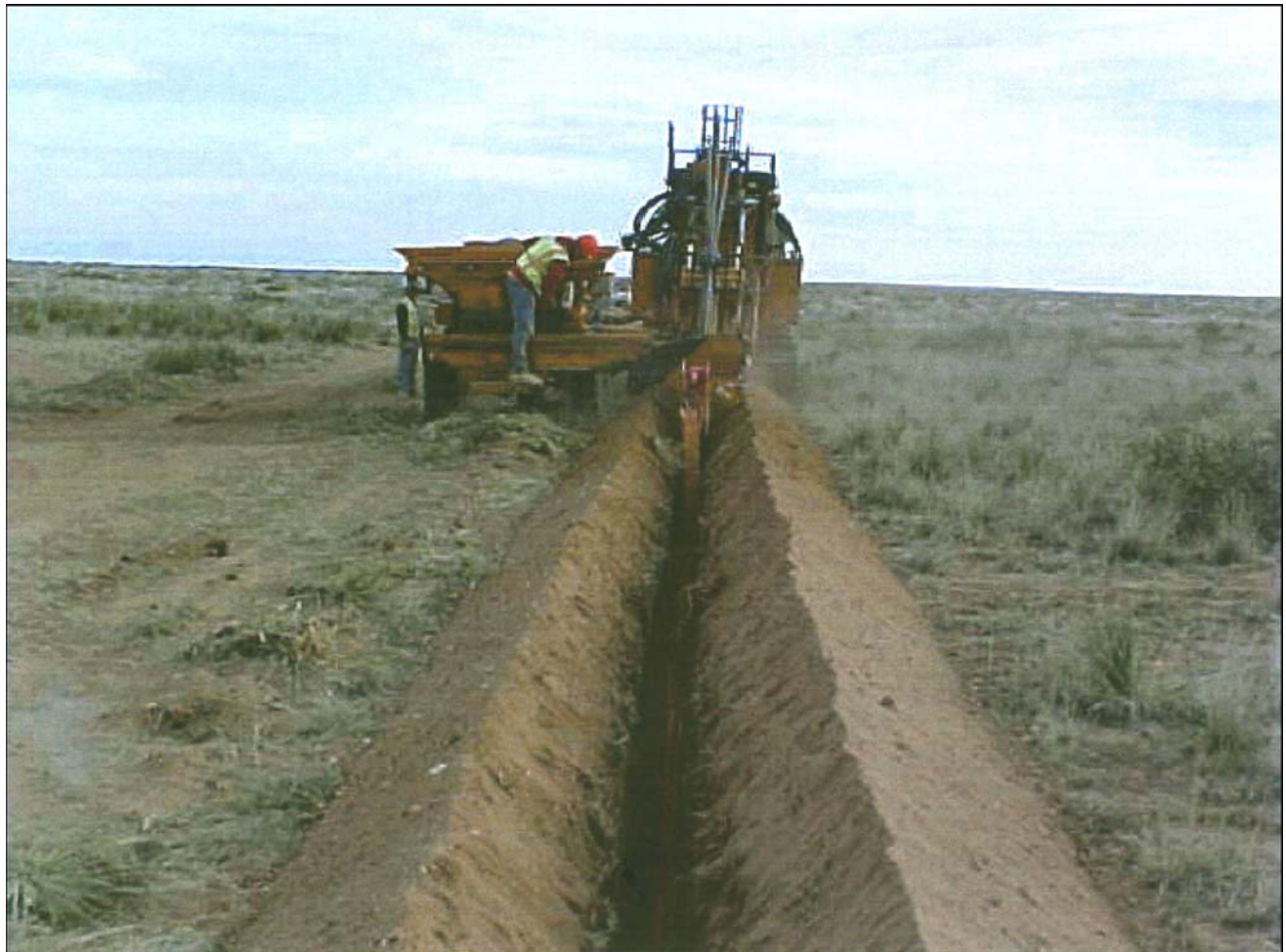
Figure 6-3 Typical trenching machine for installing the underground electric cable system
