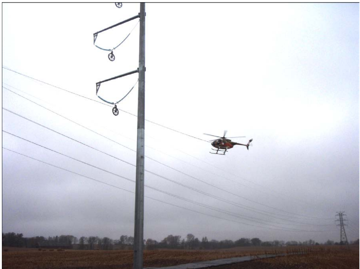
Figure Vol. 2-31 Wire stringing with a helicopter
