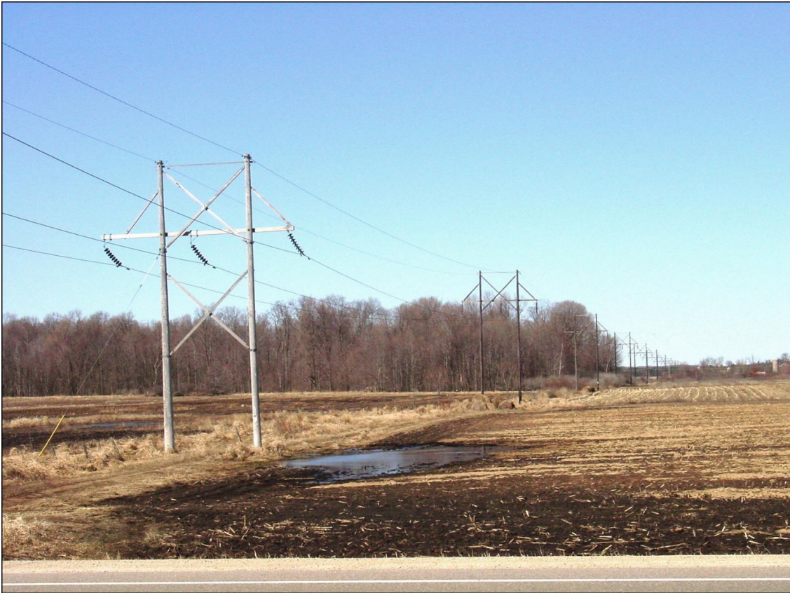
Figure Vol. 2-8 Typical two-pole H-frame structures (Image is for illustration purposes only and are not the actual structures proposed for the Badger-Coulee project.)
