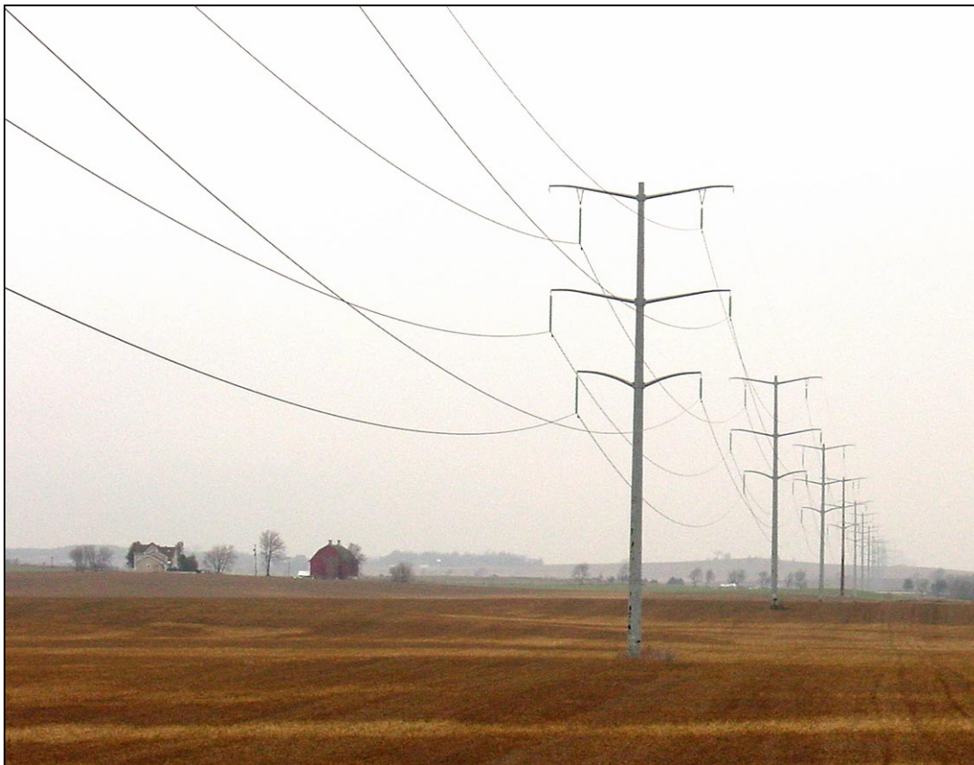
Figure Vol. 2-9 Typical single-pole double circuit structures (Image is for illustration purposes only and are not the actual structures proposed for the Badger-Coulee project.)
