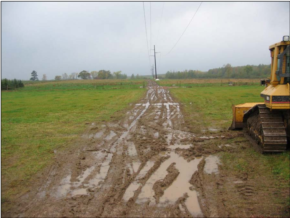
Figure Vol. 2-32 Minor soil rutting in pasture land
