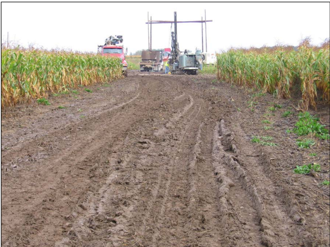
Figure Vol. 2-33 Rutting of topsoil in cropland – no soil mixing
