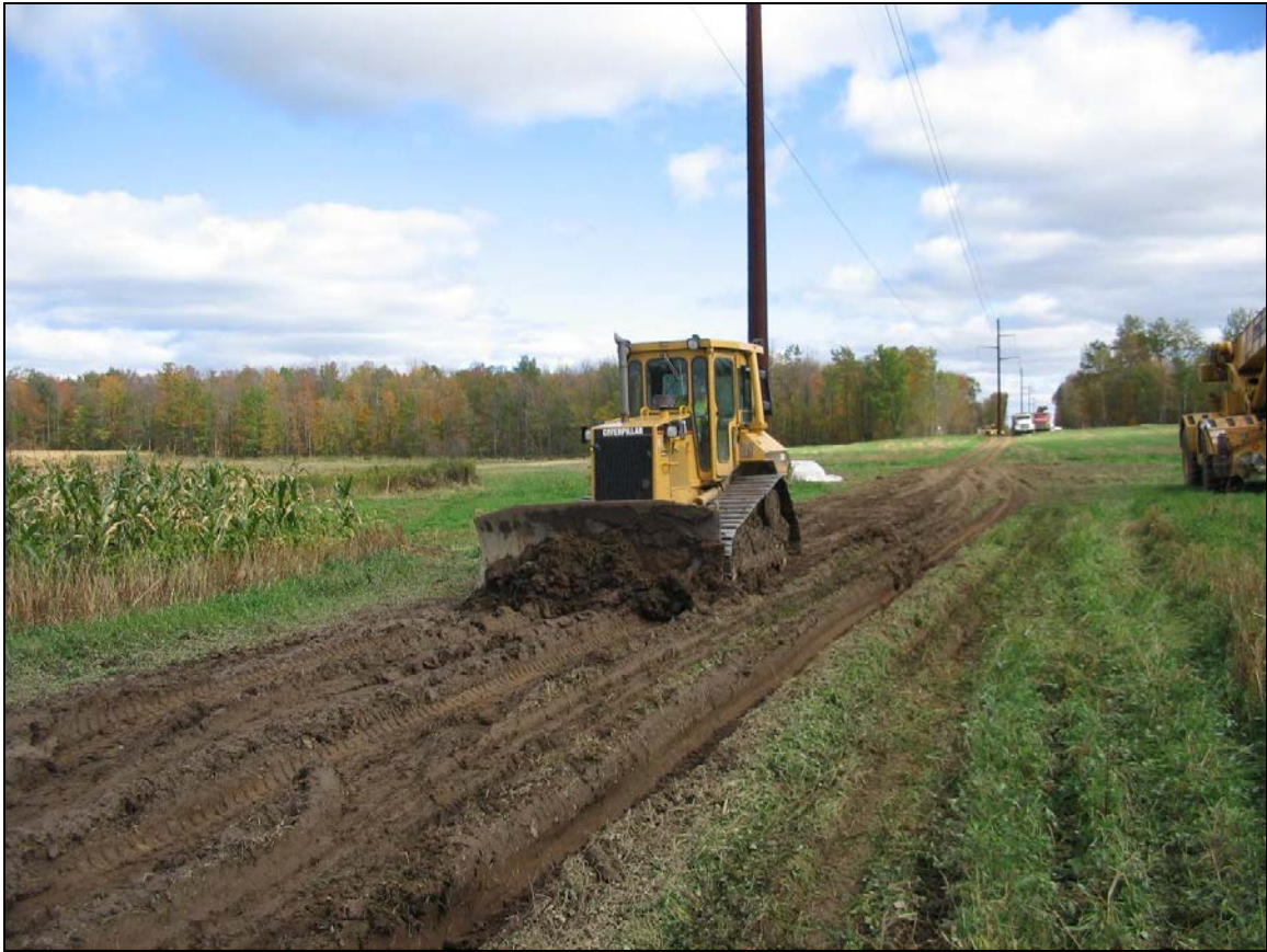
Figure Vol. 2-34 Ruts being smoothed with blade
