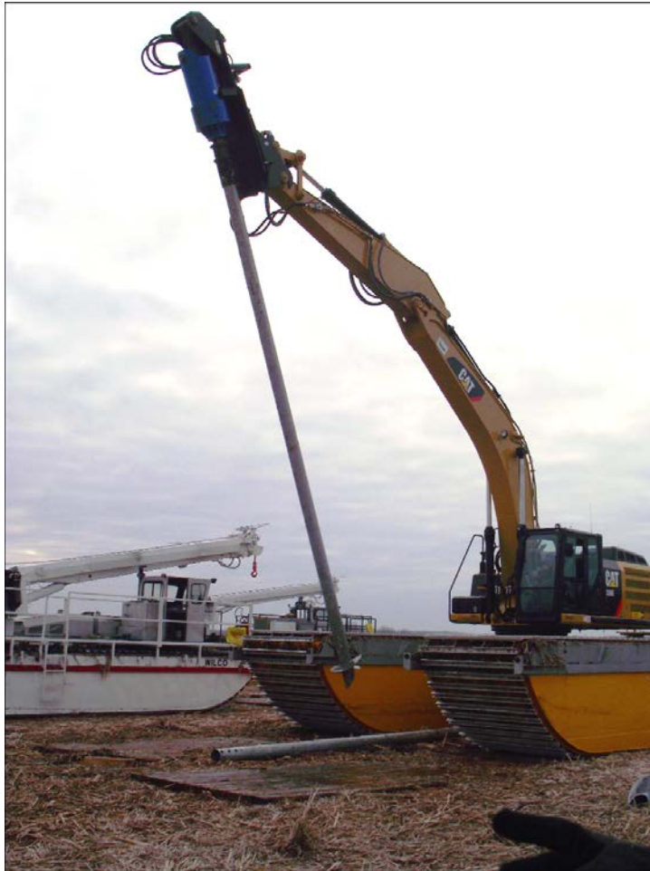
Figure Vol. 2-26 Installation of a helical pier foundation in a wetland with a marsh buggy
