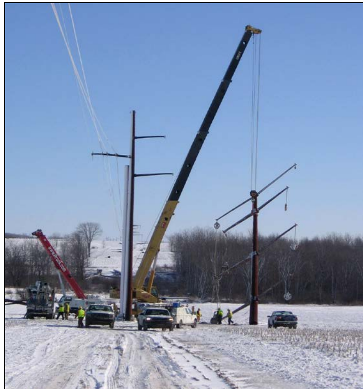
Figure Vol. 2-27 Installing the top section of the tower
