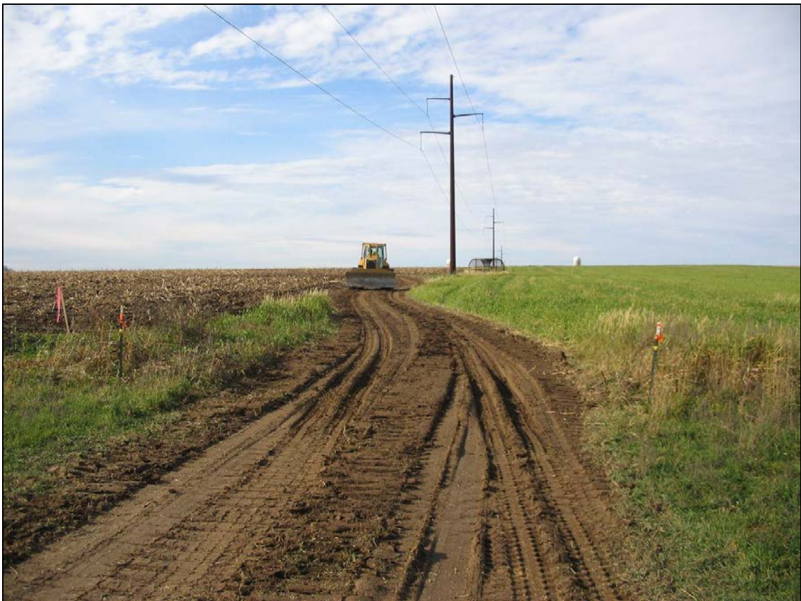
Figure Vol. 2-35 Smoothing out ruts by backblading with a dozer
