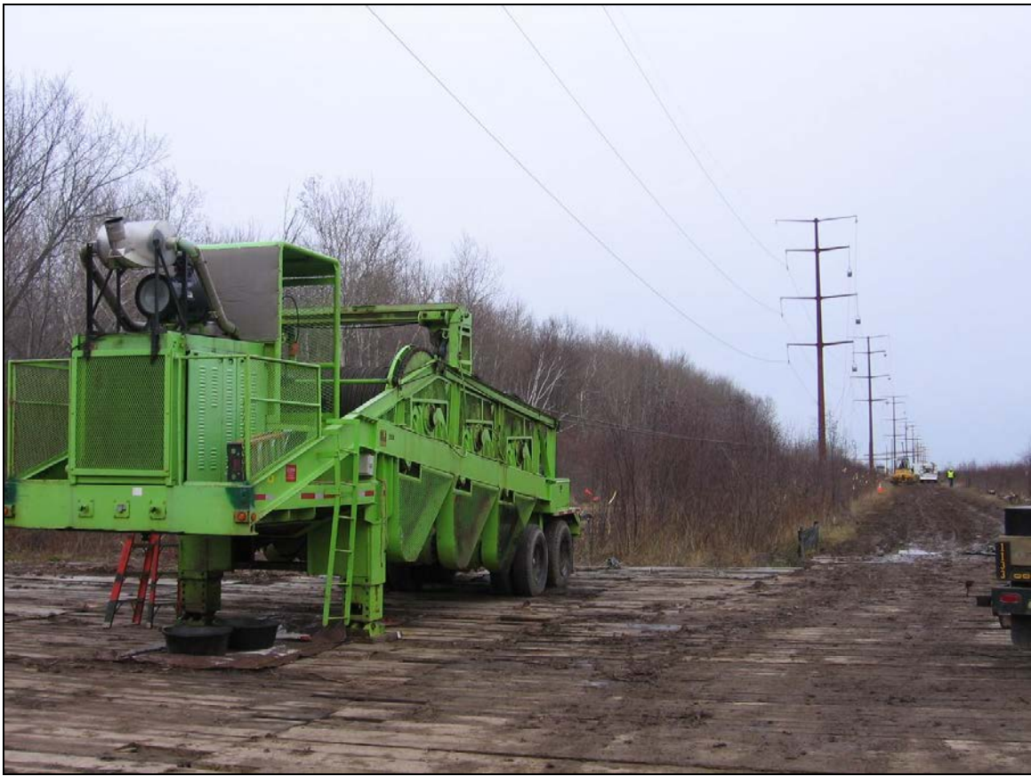
Figure Vol. 2-30 Pulling cable through structure arms
