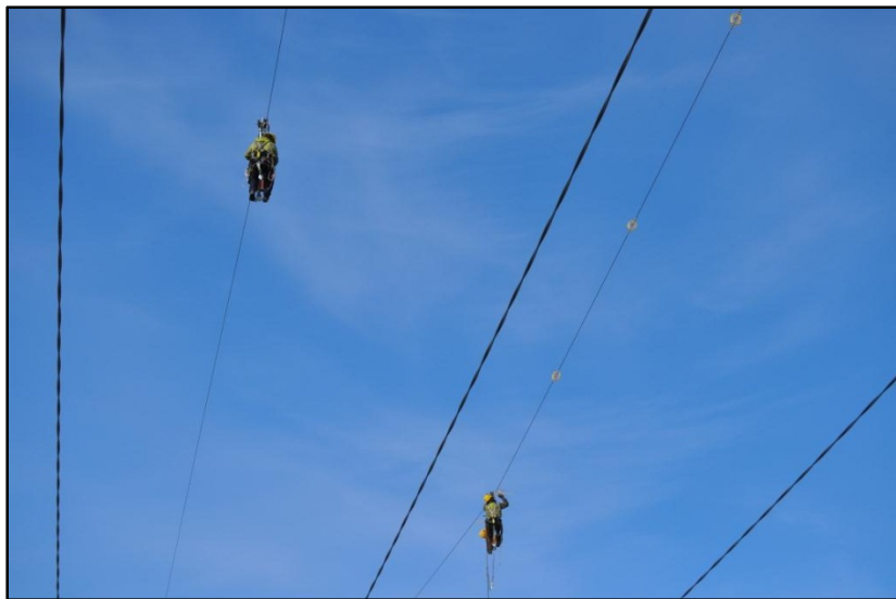
Figure 3. Swan Flight Diverters being installed on overhead shield wire of 345 kV transmission line. Note visibility and diameter difference between braided conductor wire and shield wire.
