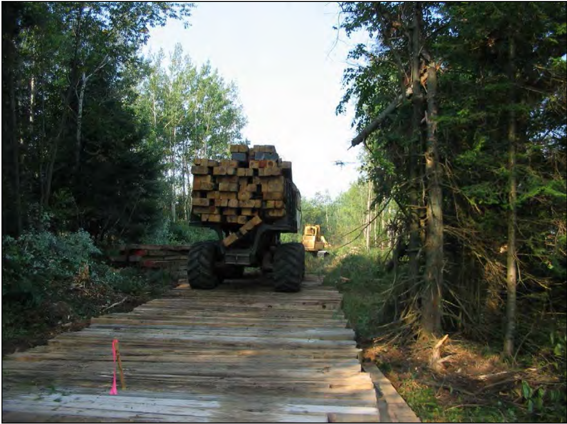
Figure Vol. 2-40 Timber mats being placed in wooded wetland
