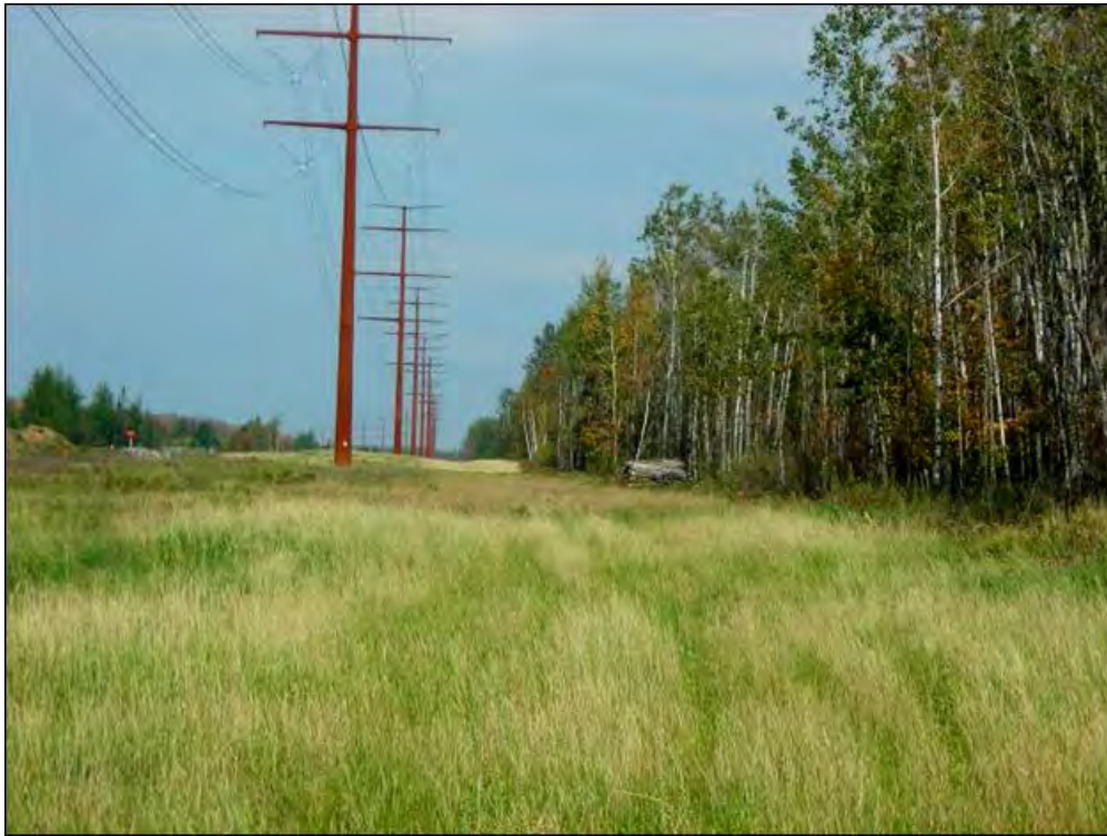
Figure Vol. 2-24 Upland ROW seeded with oats and rye grass for quick soil stabilization while native vegetation re-establishes
