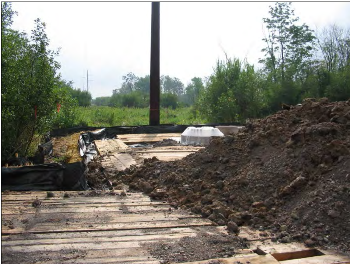
Figure Vol. 2-15 Structure location in wetland – matted work platform, foundation, spoil pile (to be removed), and erosion control
