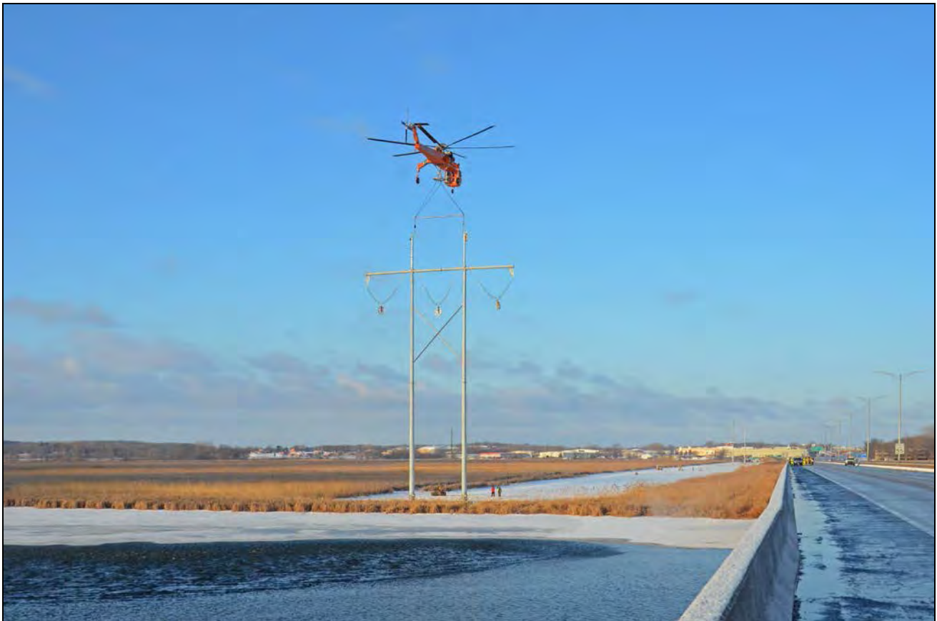
Figure Vol. 2-29 Helicopter setting tower on foundation
