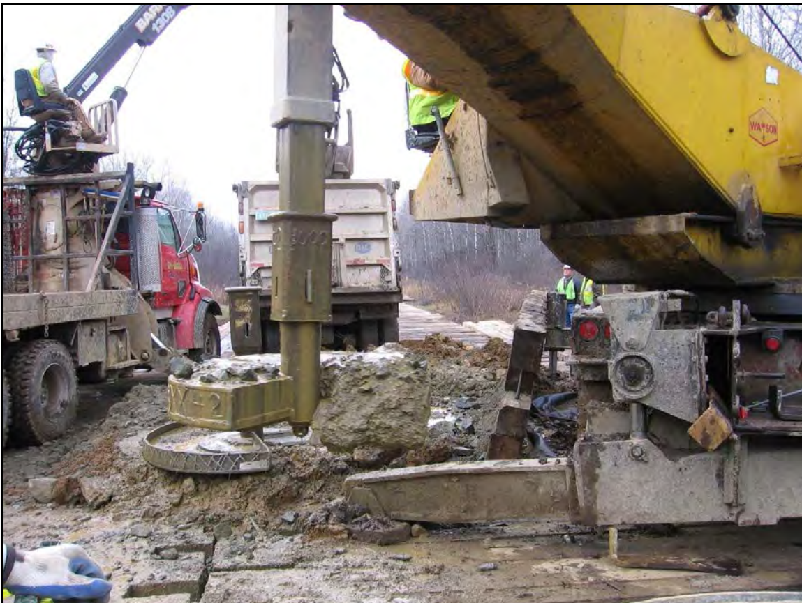
Figure Vol. 2-19 Augering rocky subsoils
