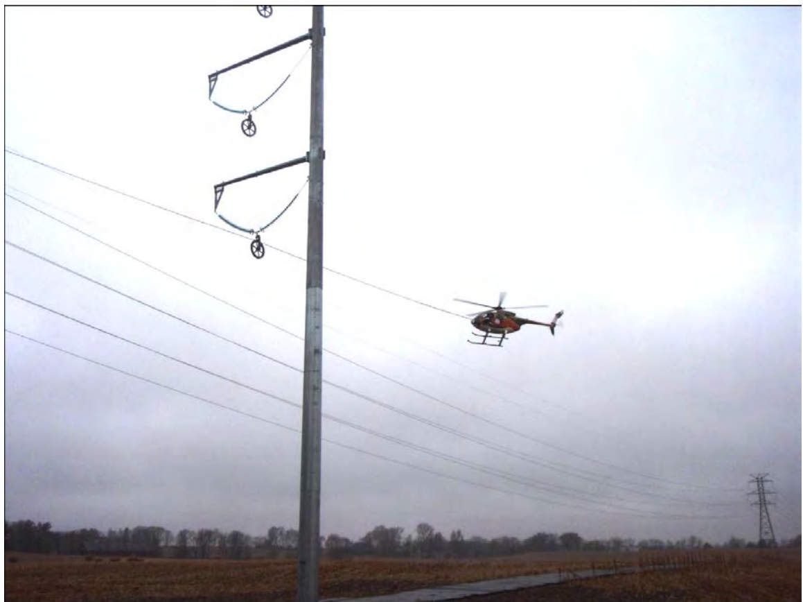
Figure Vol. 2-31 Wire stringing with a helicopter
