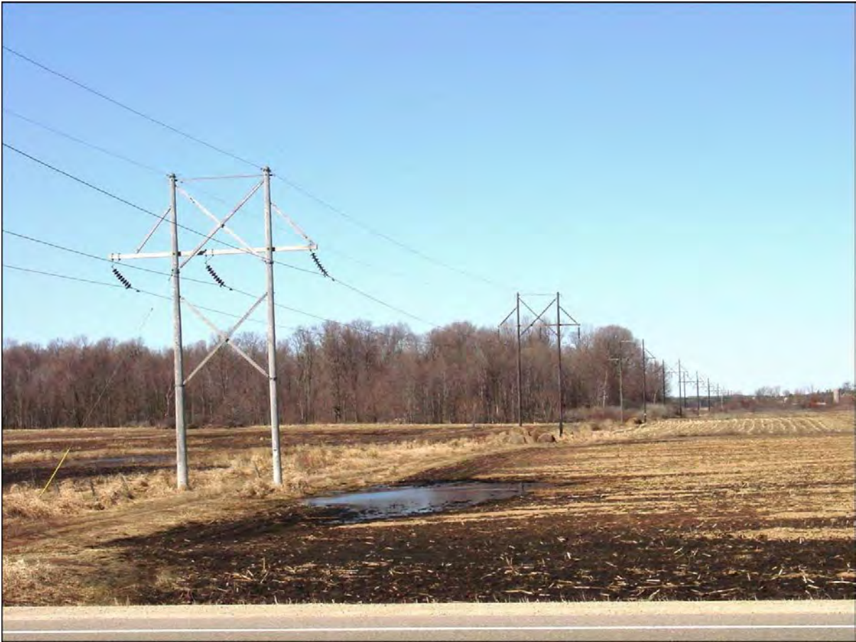
Figure Vol. 2-8 Typical two-pole H-frame structures
