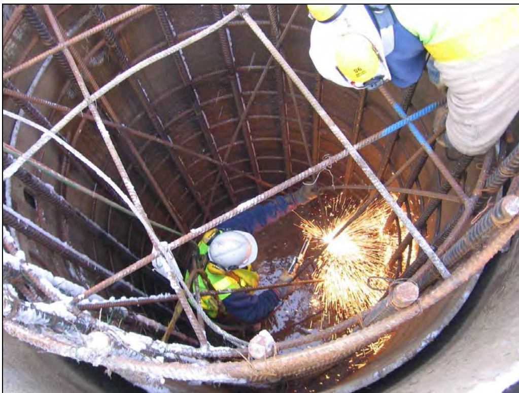
Figure Vol. 2-21 Final rebar work in preparation for concrete pour
