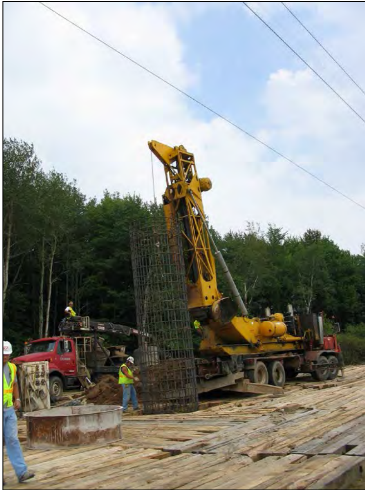
Figure Vol. 2-20 Placing foundation cage inside the excavated hole
