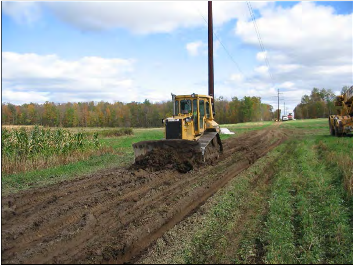
Figure Vol. 2-34 Ruts being smoothed with blade
