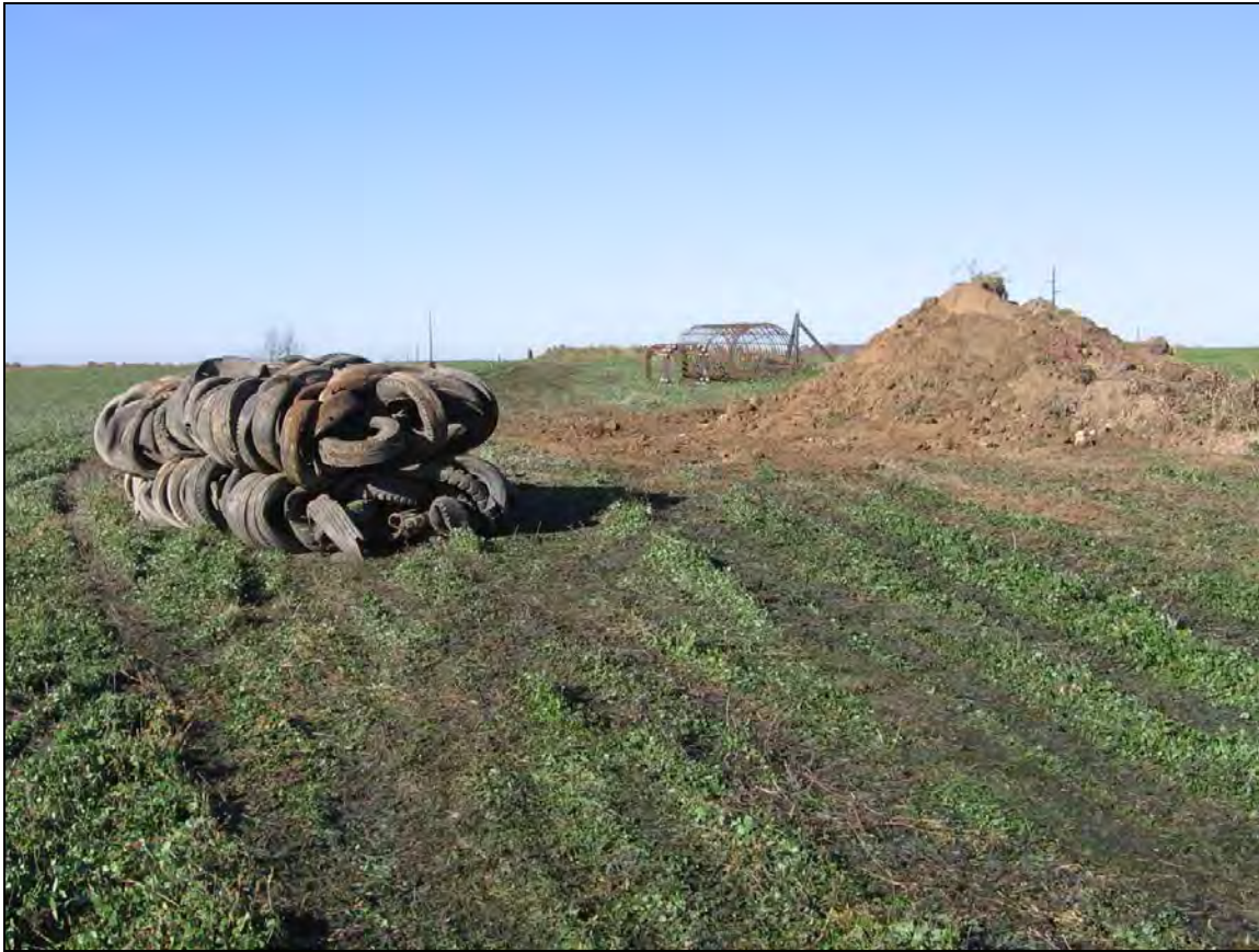
Figure Vol. 2-18 Blasting mats and post-blast soil/rubble pile
