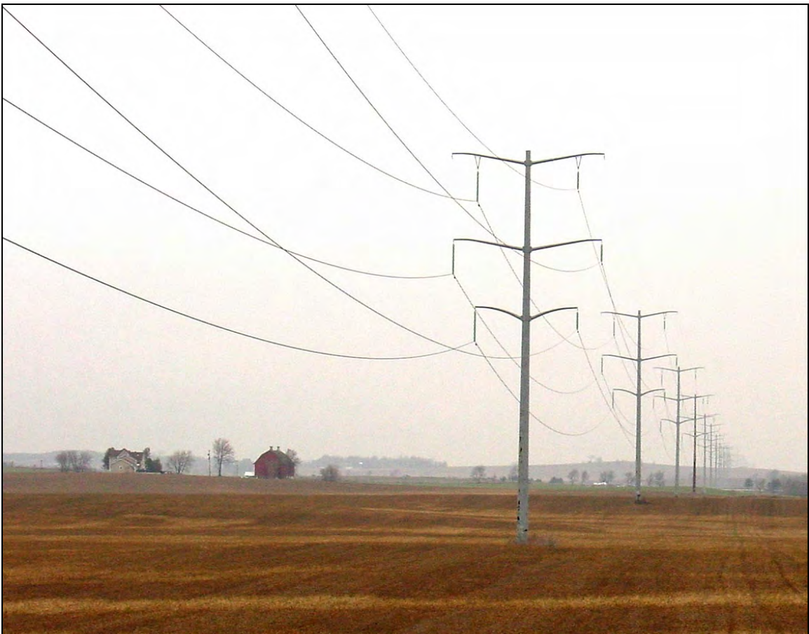
Figure Vol. 2-9 Typical single-pole double circuit structures
