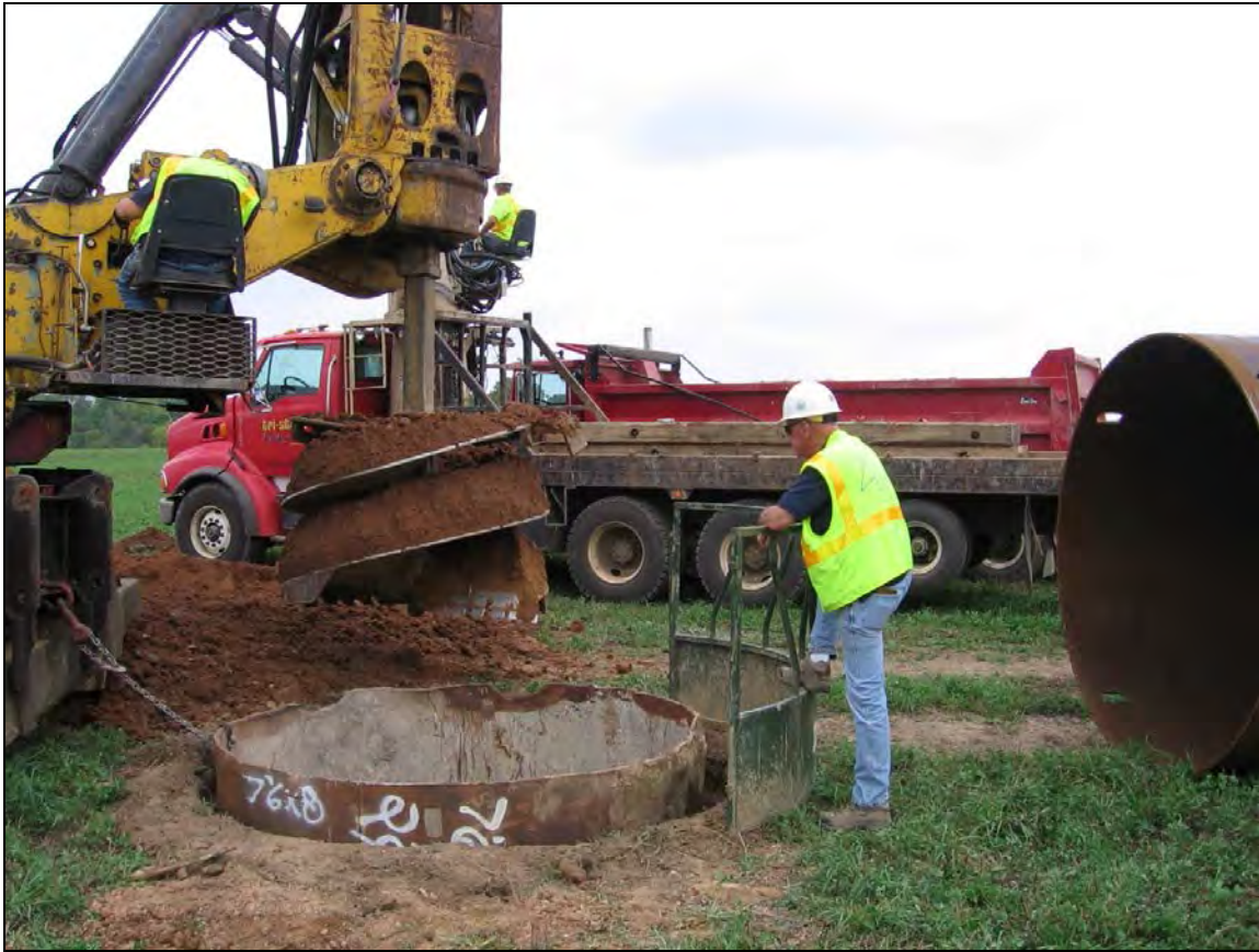
Figure Vol. 2-14 Augering a foundation excavation in dry upland soils
