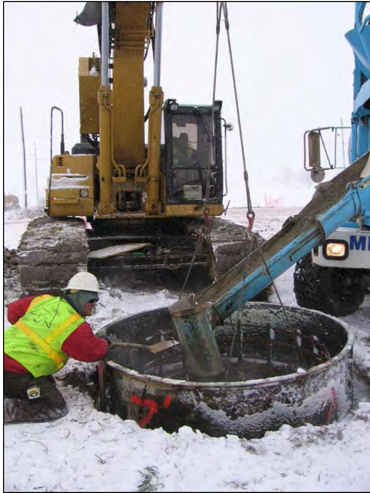
Figure Vol. 2-22 Pouring the concrete foundation
