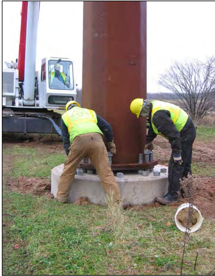
Figure Vol. 2-28 Bolting tower to concrete foundation
