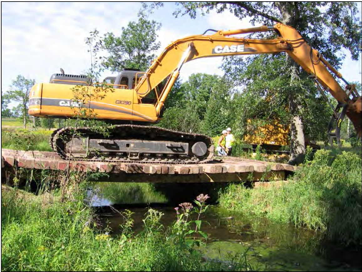
Figure Vol. 2-38 Timber mat equipment bridge at stream crossing
