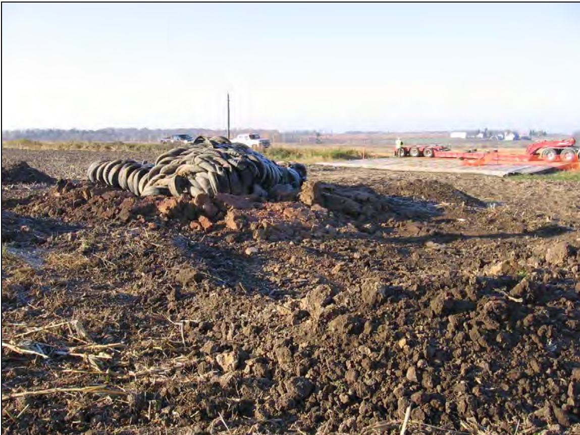
Figure Vol. 2-17 Prepared blast location – topsoil stripped and stockpiled off to side prior to blast and blasting mats in place
