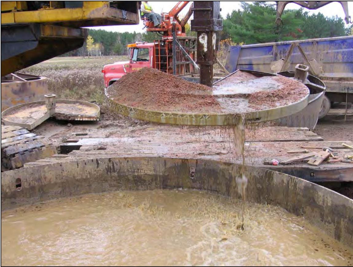
Figure Vol. 2-16 Augering in unconsolidated material (i.e gravel) – flooding of the excavation is necessary to prevent the sides from collapsing
