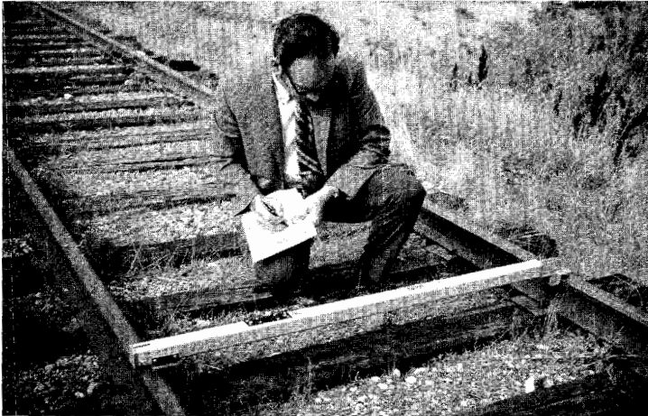
Typical staff inspection of track gauge and crossing elevation
