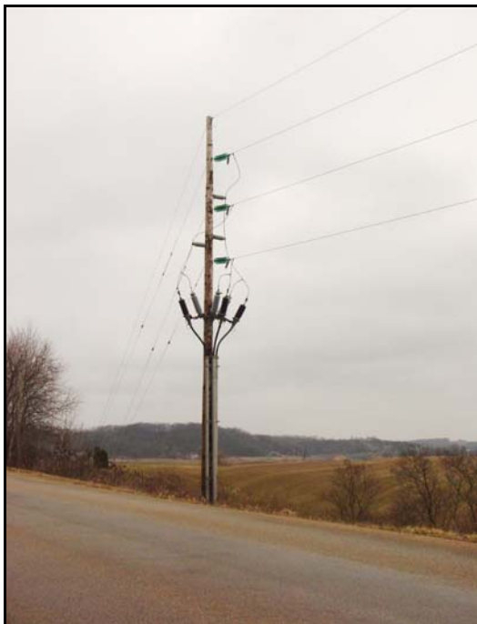
Figure 5 138 kV Underground to Overhead Transition Structures
