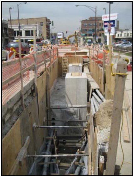
Figure 4 Vault Construction
