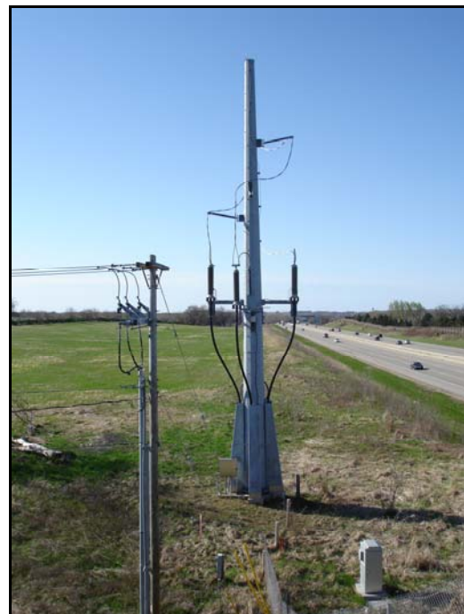
Figure 5 138 kV Underground to Overhead Transition Structures
